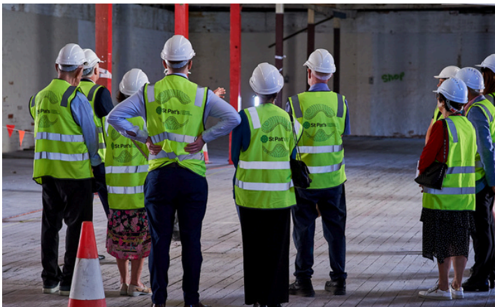
Inside of build site, redevelopment of Engagement Support Centre
